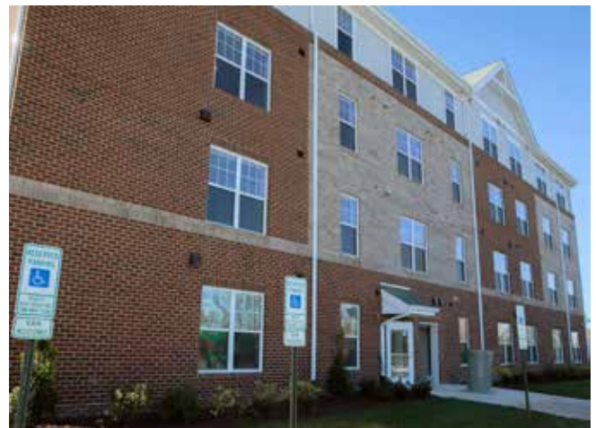
Image: Courtesy of Cedar Grove Photography LLC Nancy Hart Schrock Senseny Place in Winchester, Virginia, will provide 63 homes for seniors. The property includes a brick-and-cement panel facade inspired by the Episcopal tradition.
