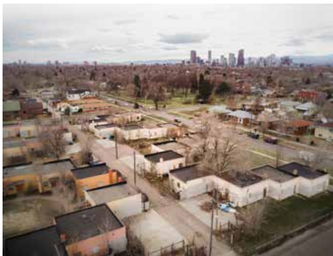
Image: Courtesy of Mile High Ministries An aerial view of the future Clara Brown Commons from the Cole neighborhood in northern Denver. Mile High Ministries is redeveloping the site using low-income housing tax credits and HOME funds.
